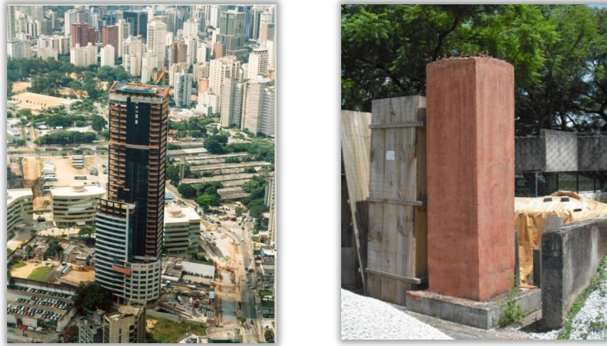
Figure 1. (a) e-Tower building, 162m high; (b) HSCC prototype replica, cast at the EPUSP laboratory yard, São Paulo, Brazil
