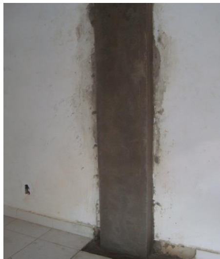
Figure 10. Final aspect of the strengthened columns.
