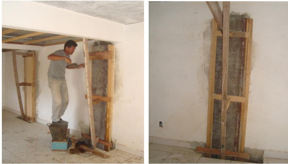
Figure 9. Concrete casting of the structural strengthening.
