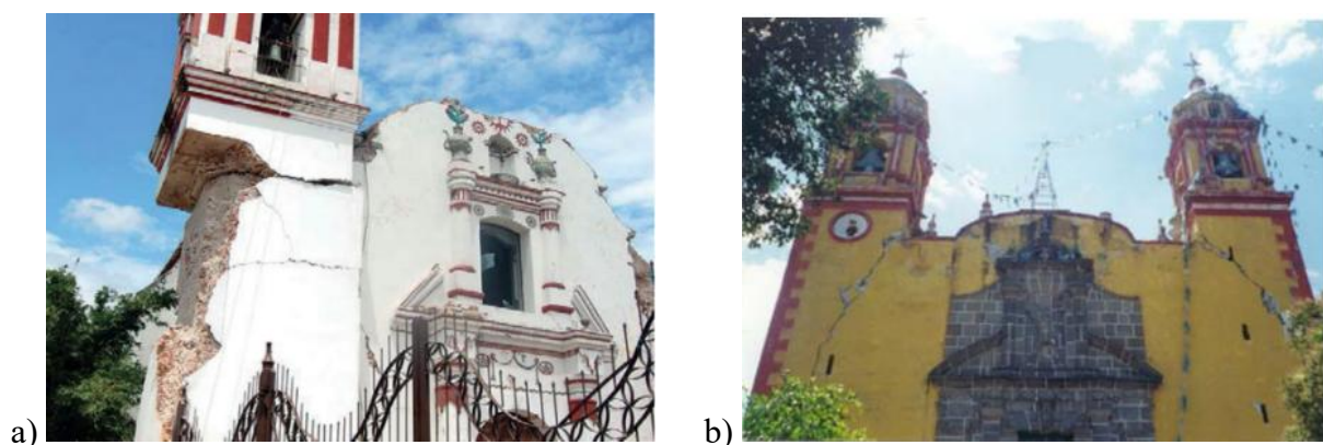
Fig. 1. Trend of deterioration and failure in bell towers attached to adjacent bodies, a) horizontal failure by earthquake with a tendency to tip over at the top by abrupt change in volume. Image taken from of the Ministry of Culture, Government of Mexico (2024), b) diagonal failure by earthquake by abrupt change in section. Image taken from: De la Torre R. O., et. al. (2004).
