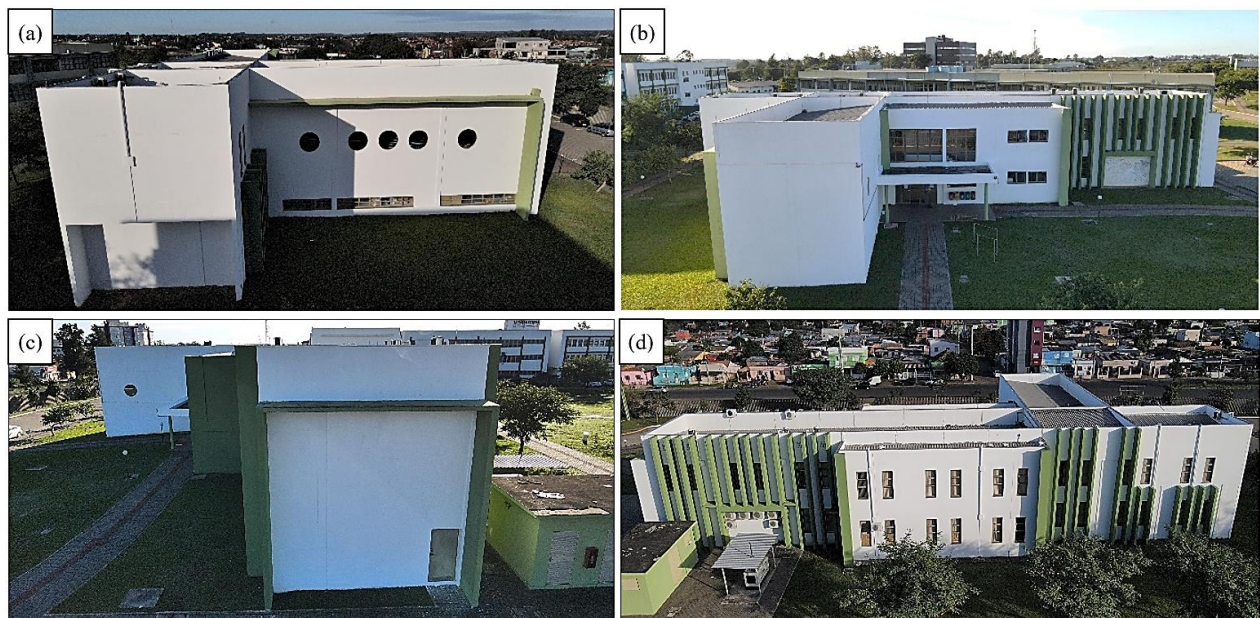
Figure 12 – North facade (a), West facade (b), South facade (c), East facade (e) after revitalization.
