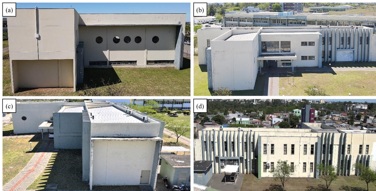
Figure 11. North facade (a), West facade (b), South facade (c), East facade (e) before revitalization
