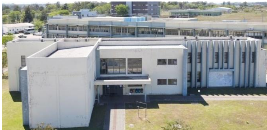
Figure 5. West facade before painting.
