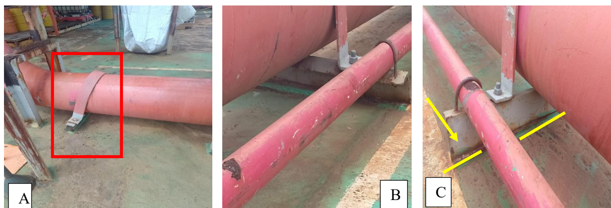
Figure 7. Deformation and crack in metal profile.
