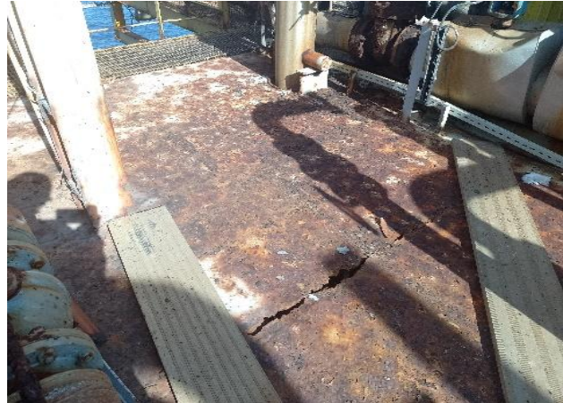
Figure 12. Effects of corrosion on metal floors and beams.
