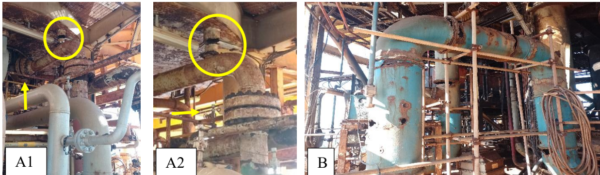
Figure 6. Damage to lines and accessories.
