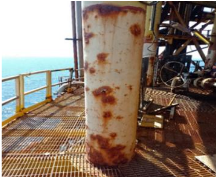
Figure 3. Alveolar corrosion.
