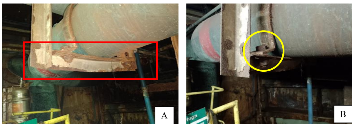
Figure 8. Screw bending and deformation of the angle bracket supporting the spool.
