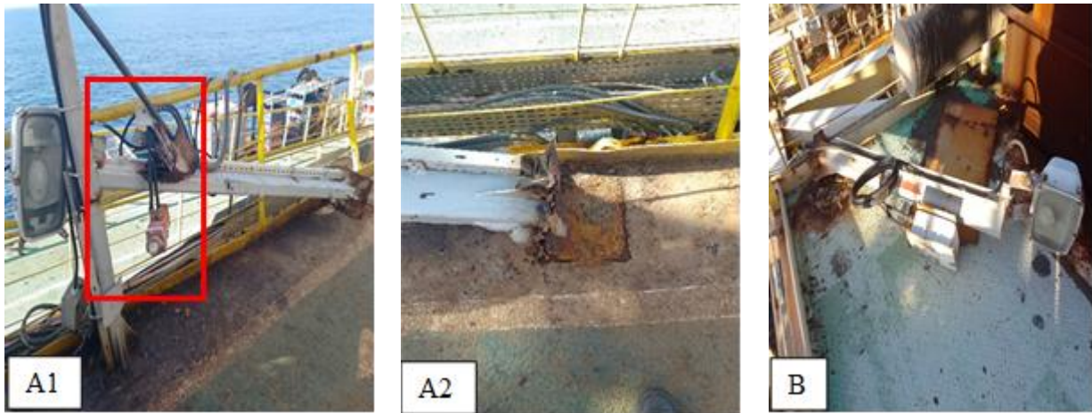
Figure 5. Collapses due to corrosion of the base of metal lighting poles.
