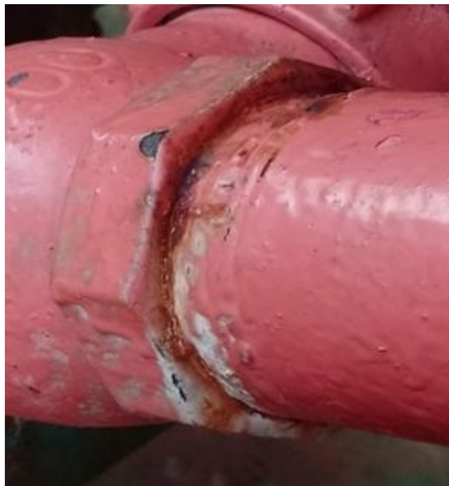
Figure 4. Corrosion in the threaded connection gap of a fire line.
