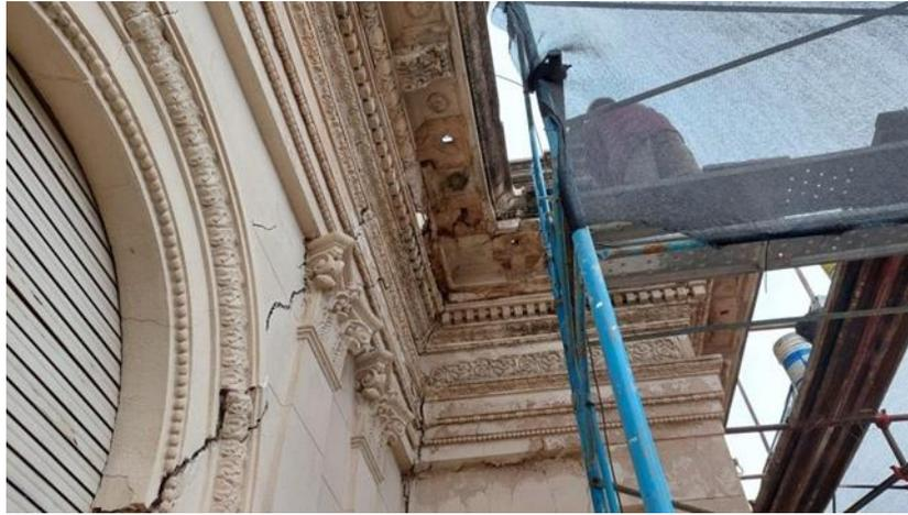
Figure 7. Detail of cracks with displacement between wall fragments.
