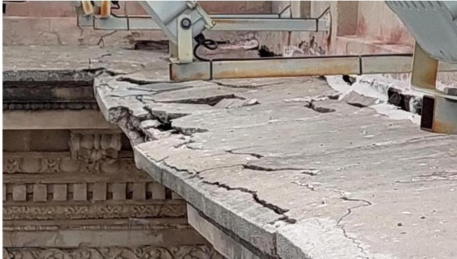
Figure 9. Deformation and breakage of the metal structure of the cornice frame.
