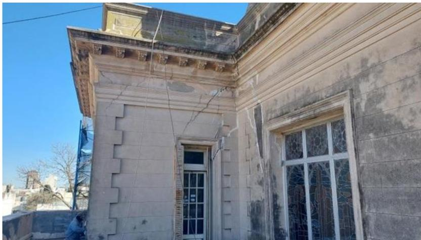
Figure 6. The differential seats caused diagonal tensile forces on the walls, resulting in the appearance of parabolic cracks perpendicular to the tensile diagonal.
