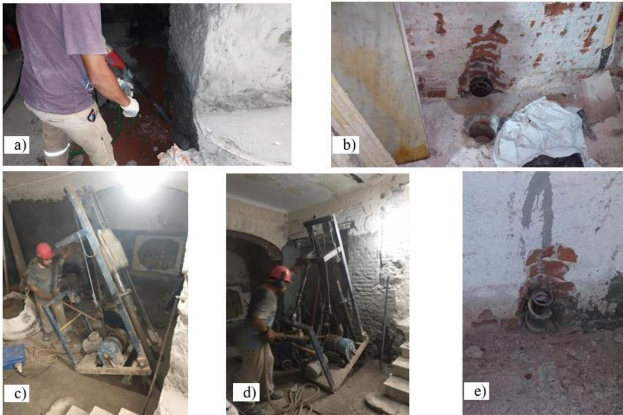
Figure 16. Detail of the intervention procedure. a) Image of diamond crown drilling. b) Photograph of the holes drilled in the masonry up to the pre-existing floor horizon. c) Photograph taken during the mechanical driving process of the micropile. (d) Photograph taken during the driving of a micropile. e) Image of the upper end of the Manessmann tube, driven, with welded abutments to increase the frictional surface against the sub-pressure slab to be executed.
