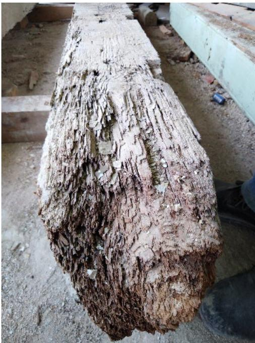
Figure 5. State of the beam heads
