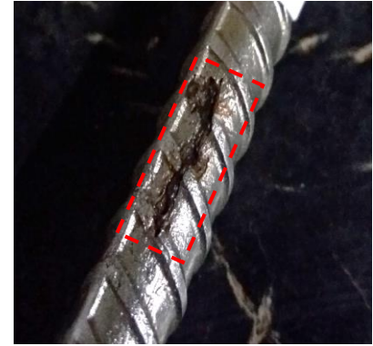
Figure 21. Mass loss from steel bars (L1).
