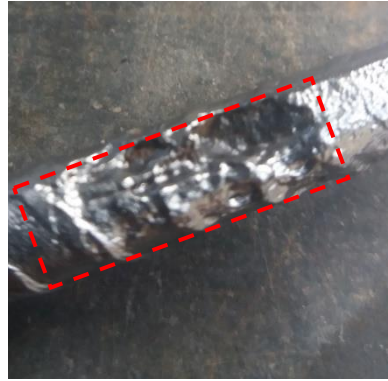
Figure 20. Mass loss from steel bars (L2).
