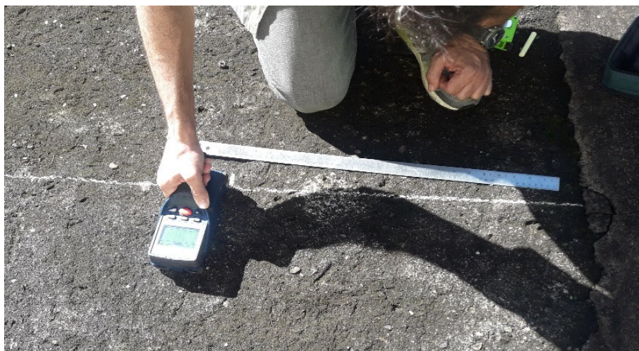
Figure 9. Carrying out the cover meter test
