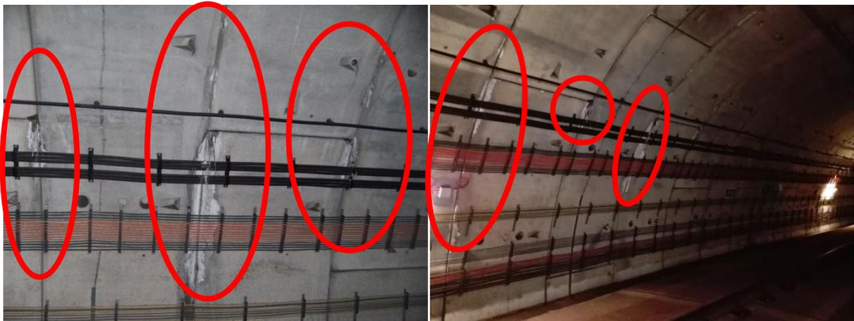
Figure 5. Filtrations (leachings of cement limes).
