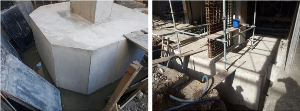
Figure 17. Detail of the visual aspect and the surface finish of concrete of reinforced pile caps.
