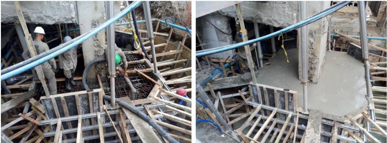
Figure 16. Detail of the concreting of reinforcement of pile cap, made with self-compacting concrete.
