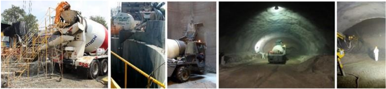
Figure 1. Primary lining placement procedure in L-12 tunnel
