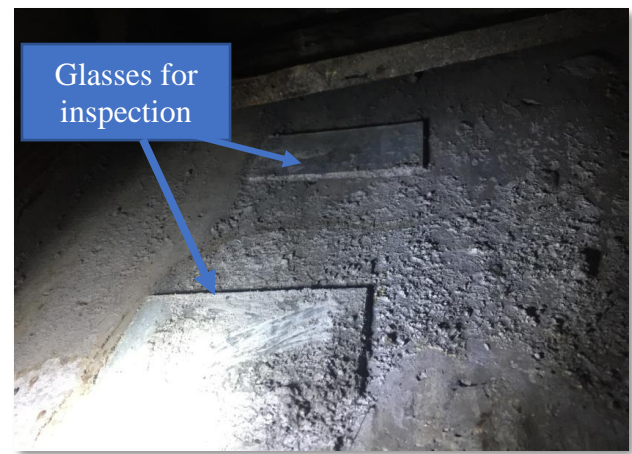
Figure 15. Interior of inspection window.
