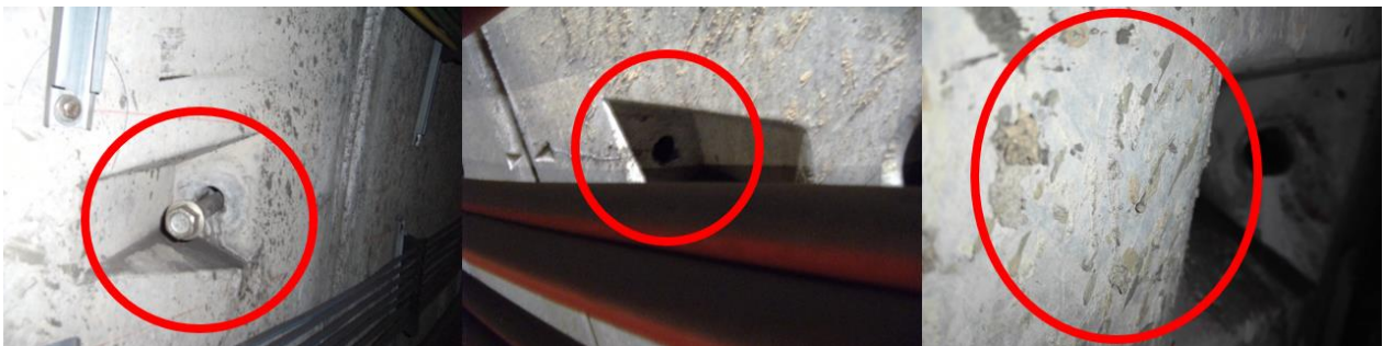
Figure 6 Roughness and clamping bolts that could affect the placement of the fiber.
