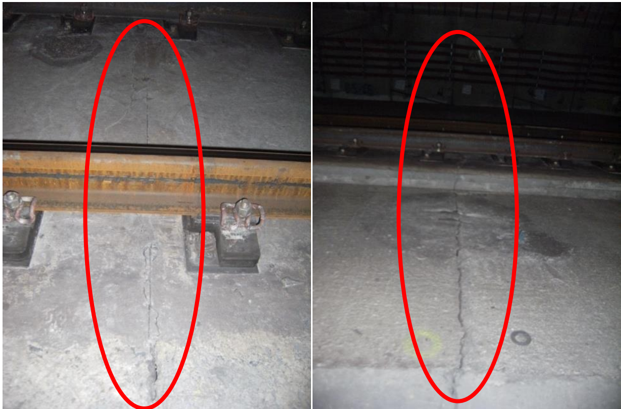
Figure 4. Joints on the track, which exist every 25m.
