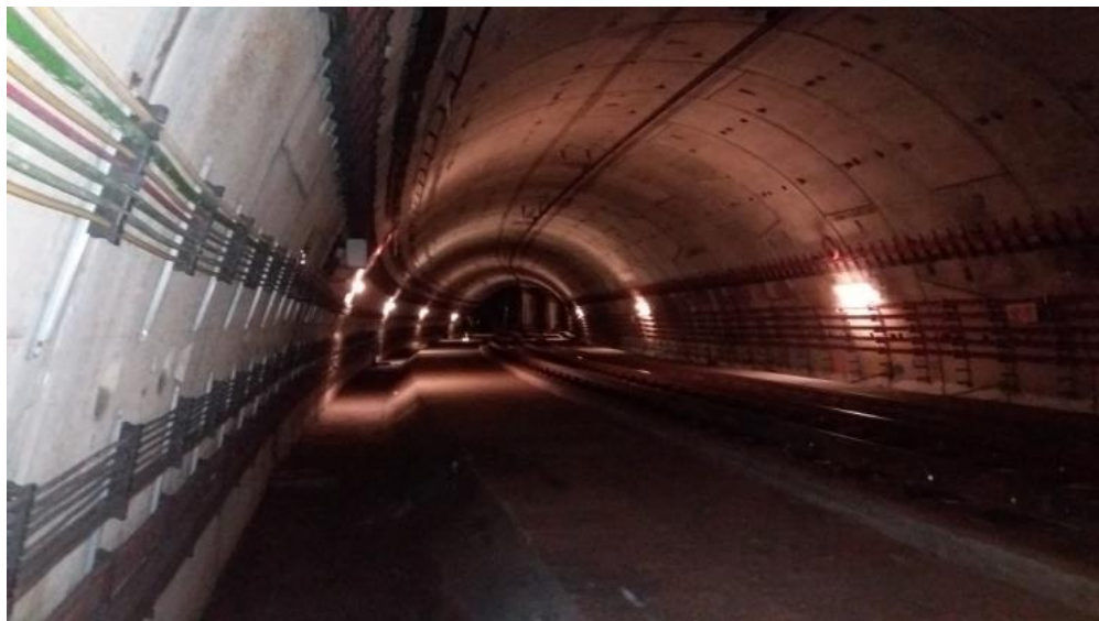
Figure 9. Overview of the tunnel in the instrumented section.
