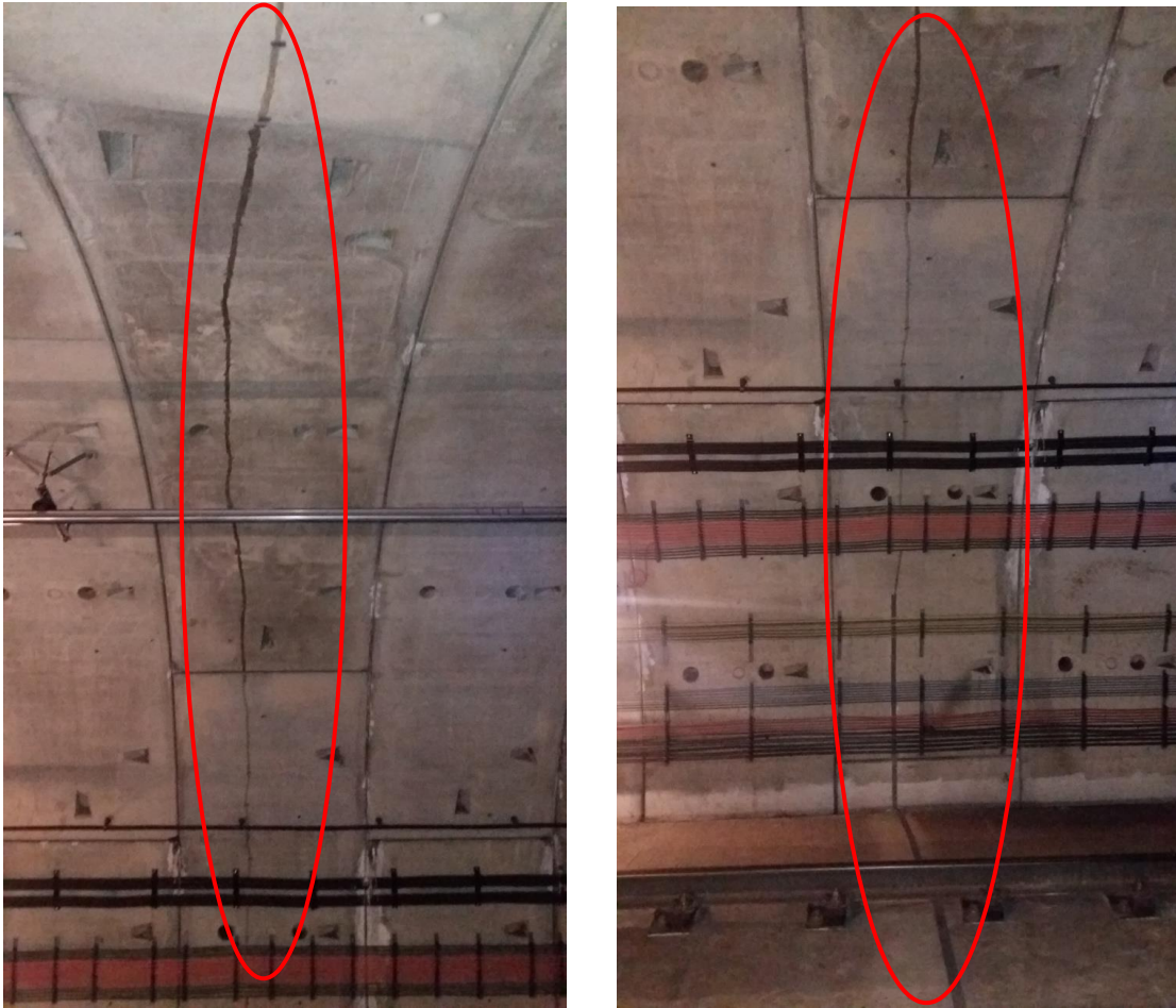
Figure 11. Optical fiber adhesion procedure on the steed of the track 2 circulation lane and in the tunnel vault.
