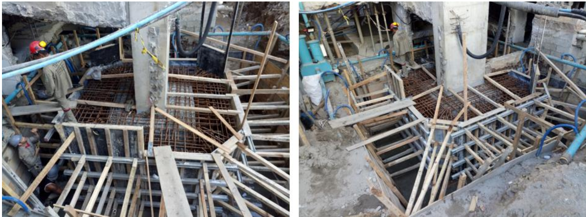
Figure 14. Detail of the formwork of structural reinforcement pile caps.
