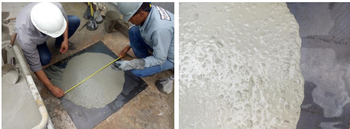
Figure 15. Visual aspect of self-compacting concrete used to reinforce structural pile caps.
