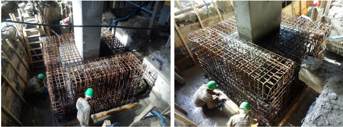
Figure 13. Detail of execution of reinforcement frame services of pile caps.
