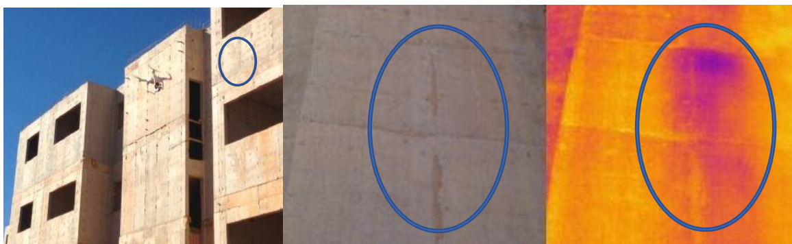
Figure 5. Inspection using an UAV integrated with a thermal camera (Nascimento, 2014)
