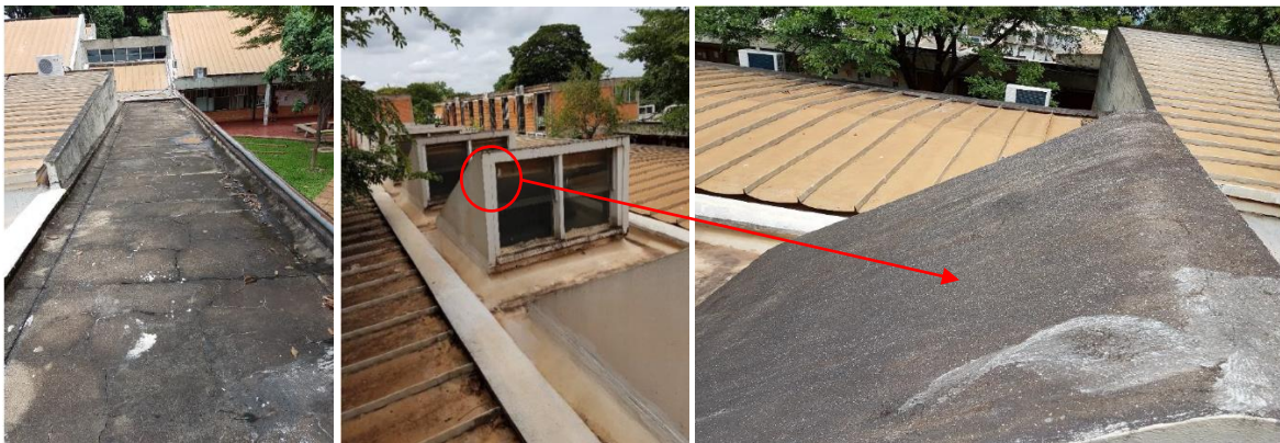
Figure 9, Figure 10 and Figure 11. Support structure without roof/skylight.
