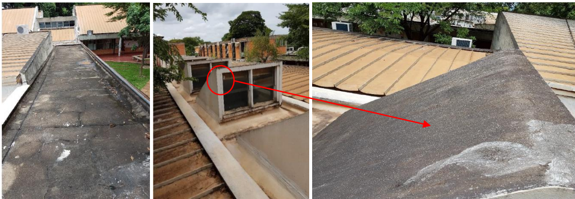
Figure 9, Figure 10 and Figure 11. Support structure without roof/skylight.
