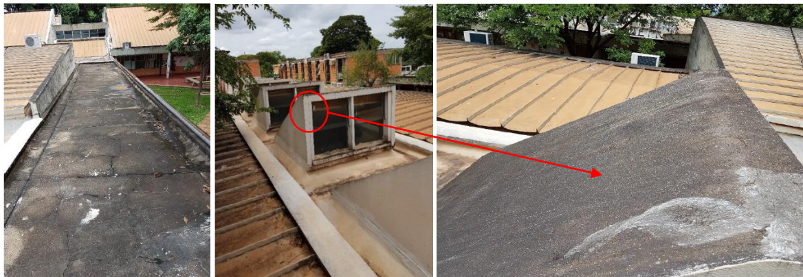
Figure 9, Figure 10 and Figure 11. Support structure without roof/skylight.
