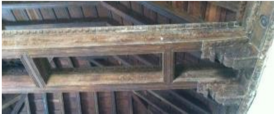
Figure 3. Tie rod beams on corbels.
