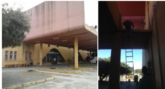
Figure 7. Location of exposure in Fragata neighborhood Fragata
