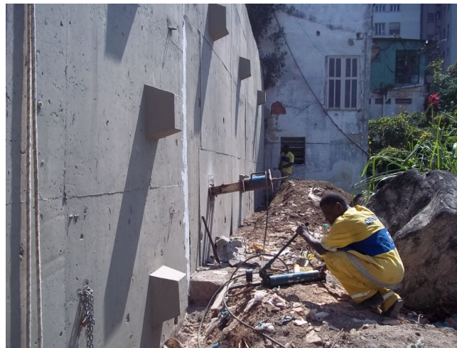
Figure 7. Residual load verification testing underway.
