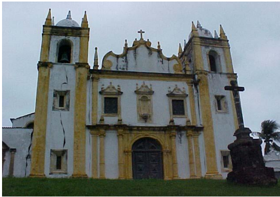
Figure 3. Structural damage to the Carmo Church in the year 2000. Source: Public Collection of Olinda.
