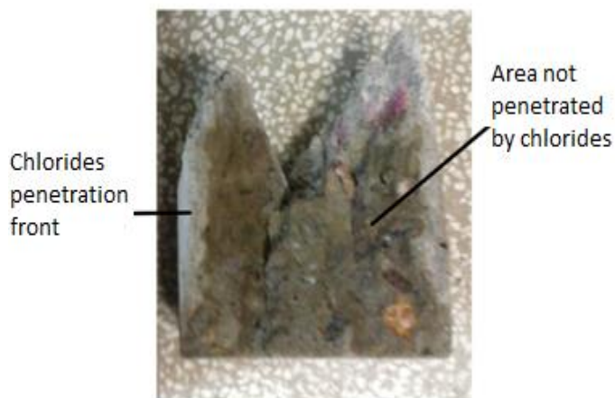
Figure 12. Example of the chlorides penetration front in the fractured simple
