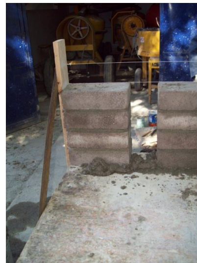
b) thread line guides for mortar joints
