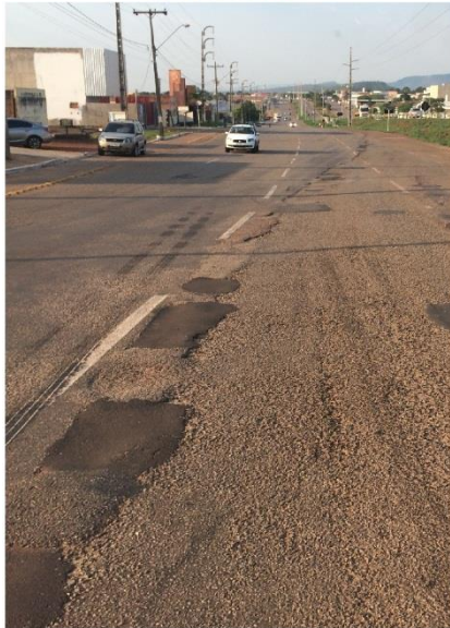
Image 7. Connection of repair.
