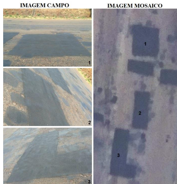
Image 10. Deep pot hole patching
