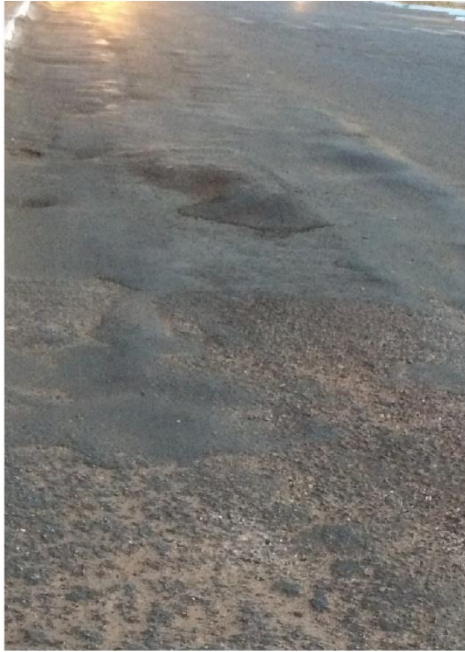
Image 6. Rutting in a stretch of heavy traffic.
