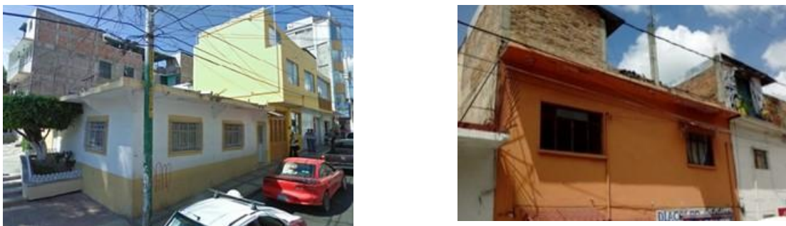
Figure 4. Housing-building of Confined Masonry
