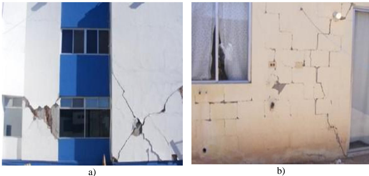
Figure 1. Masonry Walls Damage in Mexicali Earthquake, Baja California (Martínez and Martínez, 2010): a) Short Perimeter Walls, b) Housing-building Wall
