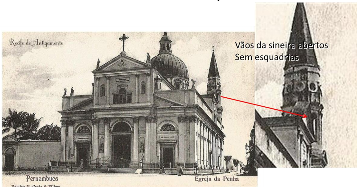
Figure 1. Historical image of the Penha-detal Basilica of the bell tower without cobogó.
