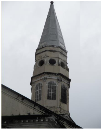
Figure 2. Current view of the tower
