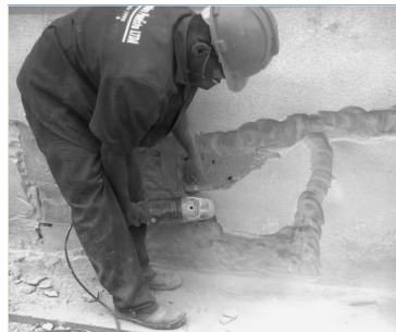
Figure 16a. Roughing process with grinding wheel
