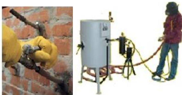
Figure 19. Injection process: placement of masters and injection through injection pump
