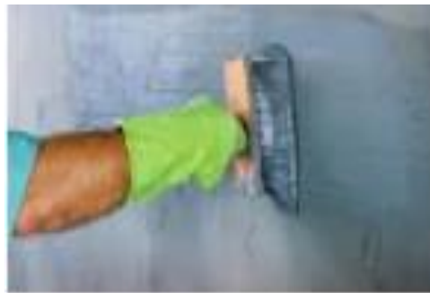
Figure 17b. Primer application as surface preparation
