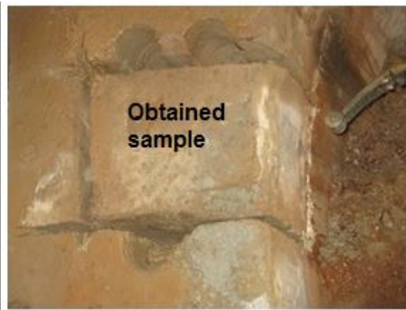
Figure 8. Sample removed from masonry sent to the laboratory.
