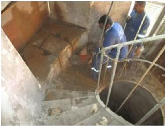
Figure 7. Sample removal process using double diamond disc.
