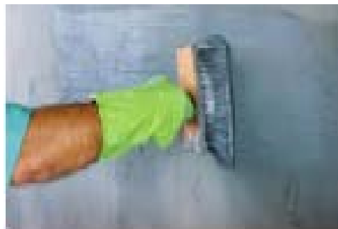
Figure 17b. Primer application as surface preparation
