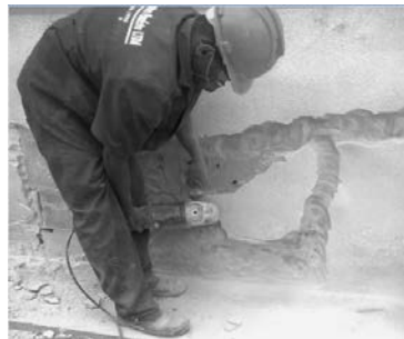
Figure 16a. Roughing process with grinding wheel
