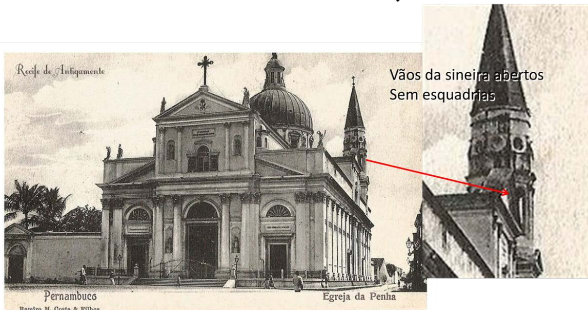
Figure 1. Historical image of the Penha-detal Basilica of the bell tower without cobogo.
