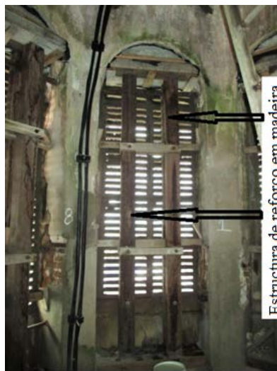
Figure 3. Reinforcement in tower columns
