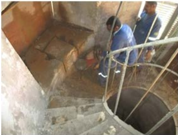
Figure 7. Sample removal process using double diamond disc.
