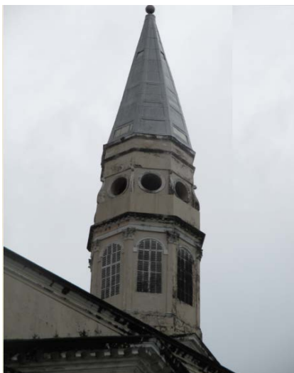
Figure 2. Current view of the tower
