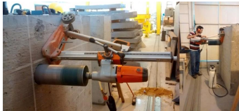
Figure 7. Drill advancement steps
