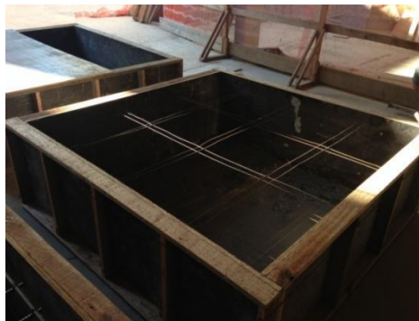
Figure 1. Molds for the concrete pouring of the wall
