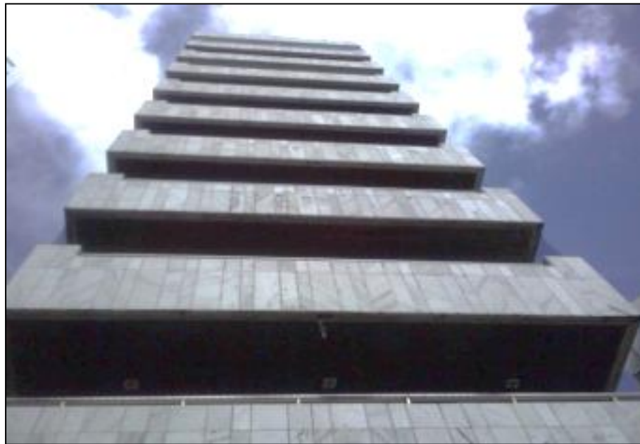
Figure 3. Eastern facade (section T1).
