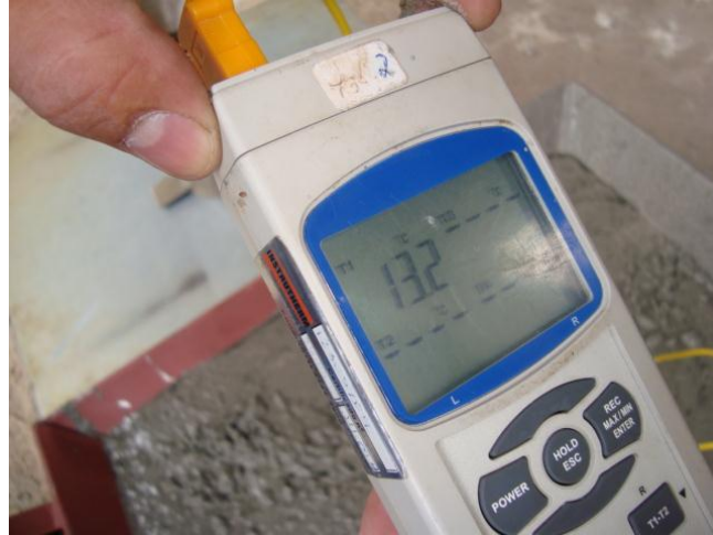
Figure 8. Fresh concrete temperature was controlled for each mixer truck by means of an immersion digital thermometer (example: 13.2°C).
