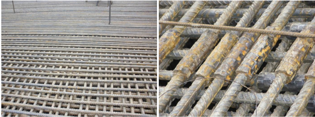
Figure 12. The superior reinforcement consisted in two double layers of 32mm rebars. SCC concrete mix was designed to pass through this reinforcement.
