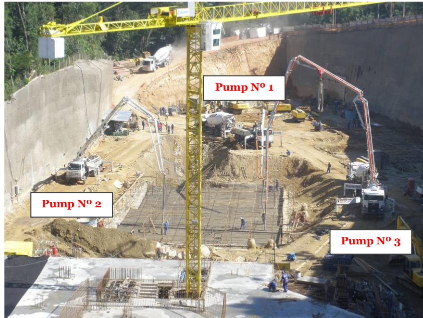
Figure 10. General view – Concrete pumps positioned.
