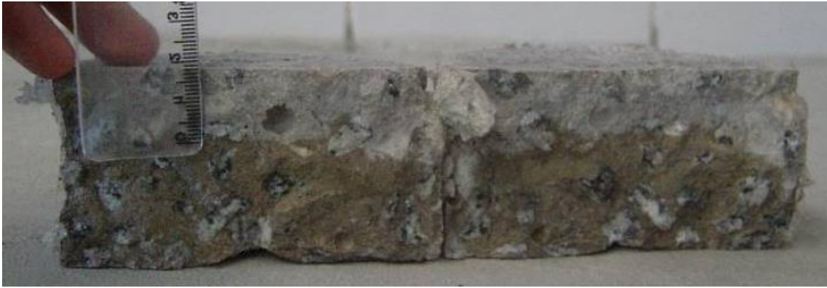
Figure 1. Potential precipitation of free chlorides (white) and combined chlorides (brown) (Medeiros et al, 2009).
